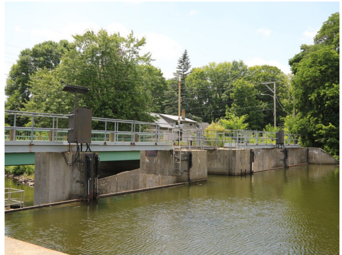
Sebasticook Lake outlet dam. Photo credit: Bowman Construction
