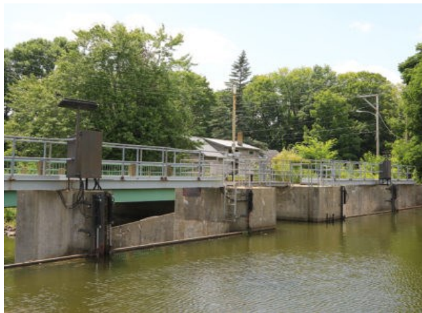
Sebasticook Lake outlet dam. (Photo credit: Bowman Constructors)
