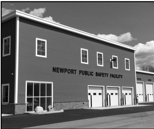
Newport's new Public Safety Building
